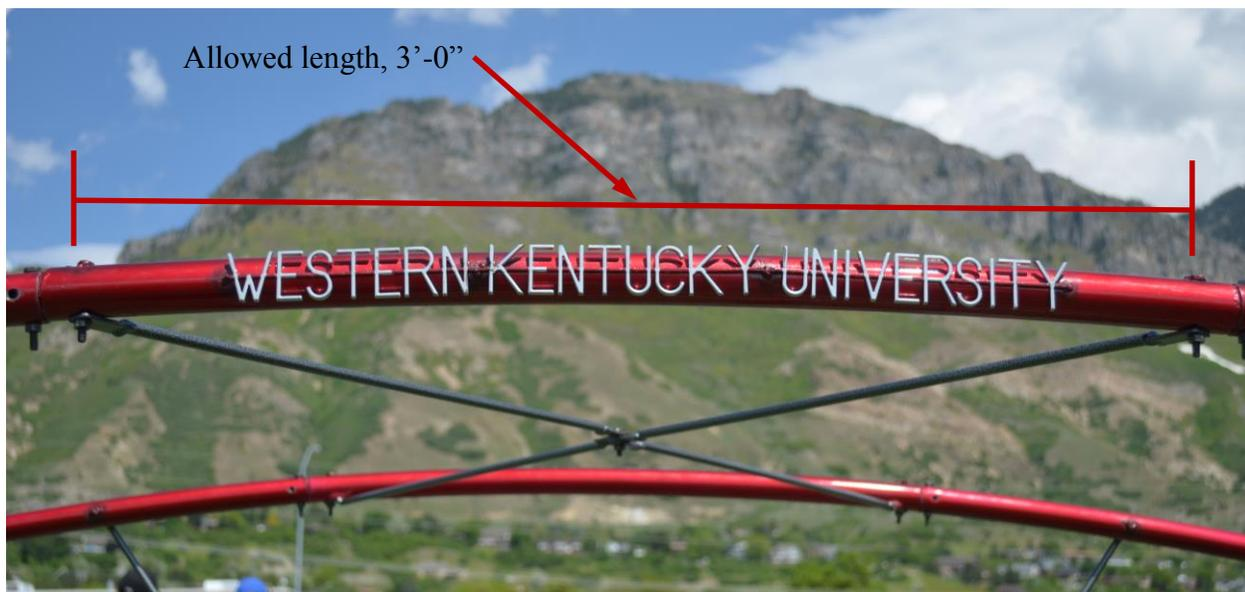
Figure 2. Center steel arch member, longer than allowed
